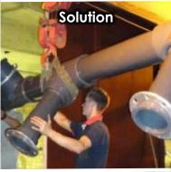
The new pipework was pre-fabricated, brought to site ready-to-install and craned into place, ensuring that the pumps and pipework could be replaced in one night so that the pool could remain fully operational during normal opening times.
